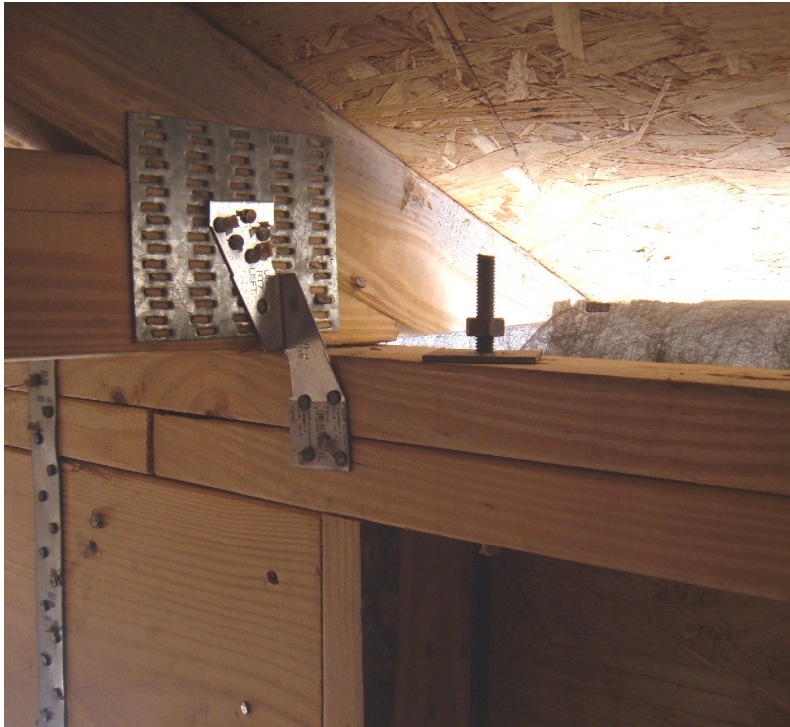
Figure 7: What was once a nut tightly secured to the bearing plate, now has a gap as wood shrinkage and dead compression occur throughout the structure.
